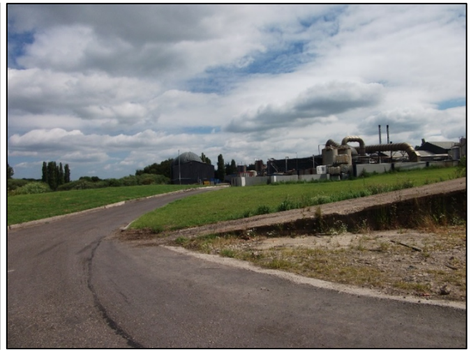
View across site looking north east
